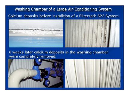
Filtersorb SP3 is successfully used in a number of applications for both residential and commercial usage. Virtually maintenance free, chemical free, and salt free, Filtersorb SP3 media water conditioners are a cost effective alternative where benefits and overall performance surpasses our competitors.
