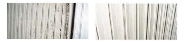
About six weeks after the installation of the Filtersorb SP3 Systems the calcium deposits were completely removed
